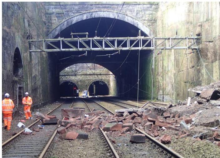
**Fig.2:** Debris lying on the track within a railway cutting, near Liverpool Lime Street station, UK. Note the potential for a catastrophic incident to occur if a service train had been passing through the cutting at the time, with line speeds of 30 and 40mph. **Source:** Railway Accident Investigation Branch, 2017.
