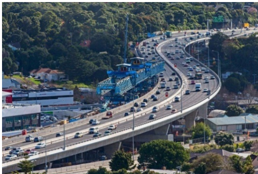
Figure 1. Aerial view of Newmarket Viaduct.
