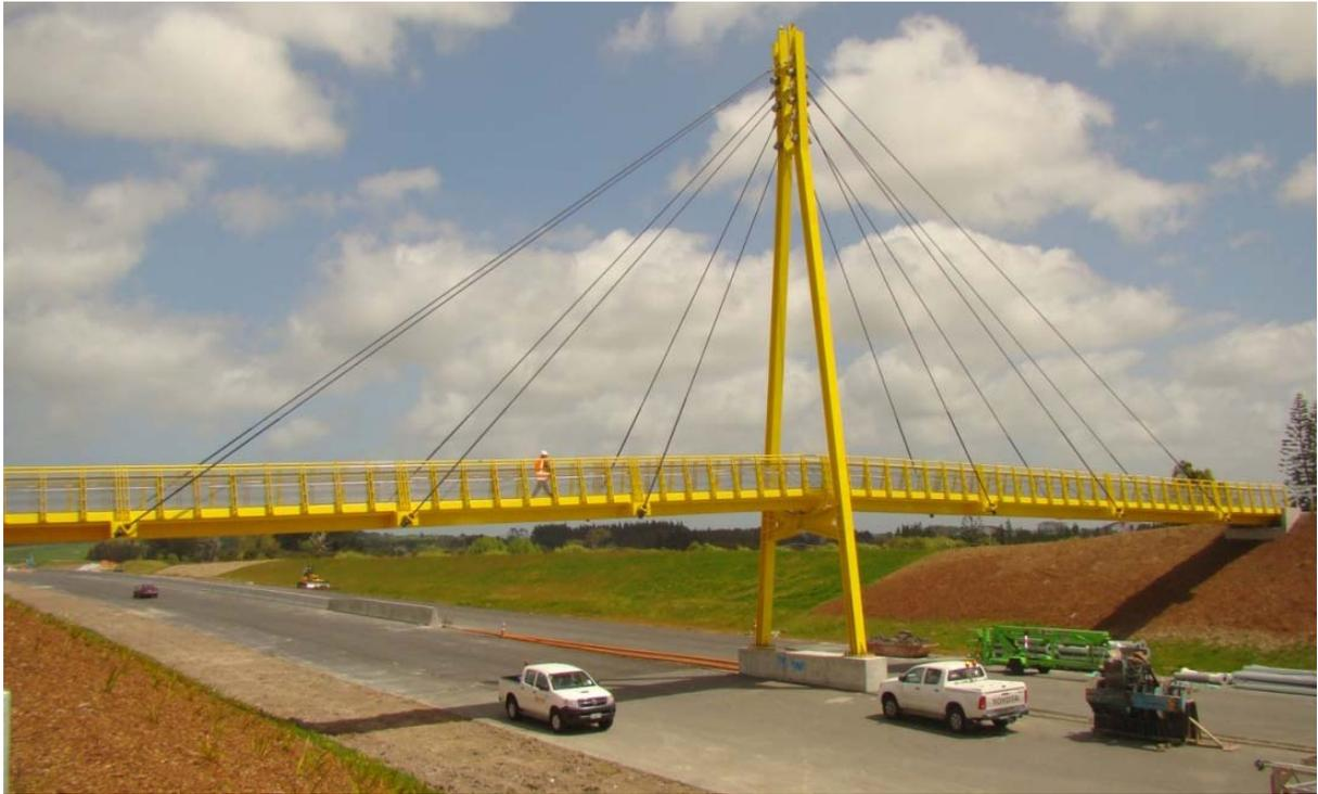
Figure 2. Full-scale cable-stayed footbridge.
